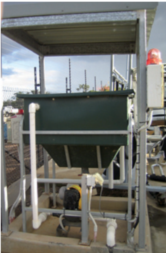
A coalescing (corrugated) plate interceptor (CPI) treats wastewater before it is discharged to the sewer.
