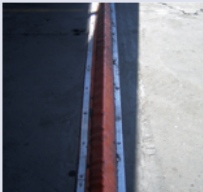
Choose the bund most appropriate for your workshop. These photographs show two types of drive-over bund.
