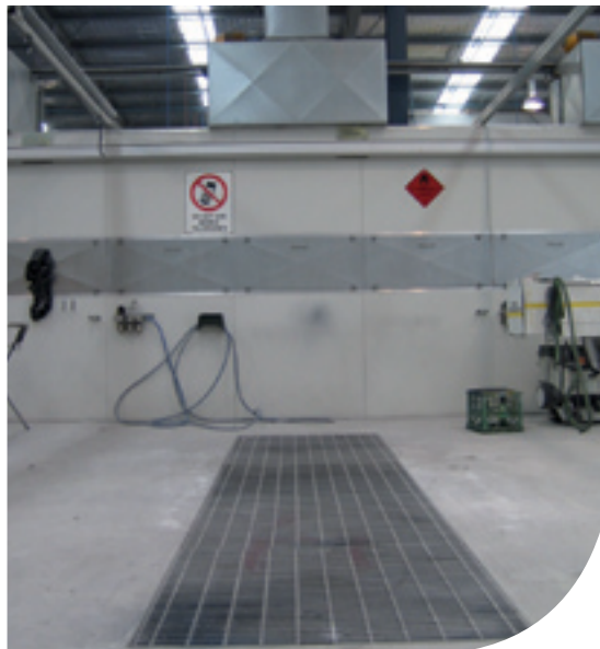
Spray booth filter in preparation area.
