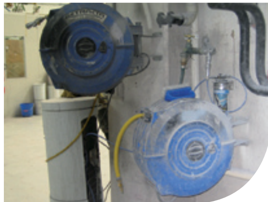
Maintain compressor hoses to avoid wasting electricity.
