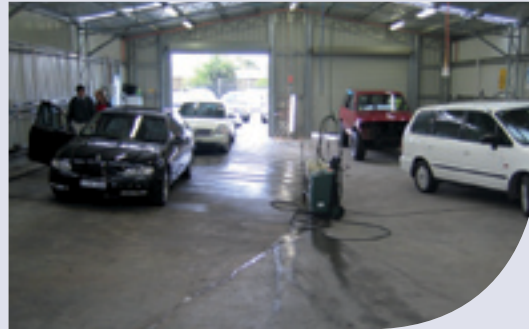
A floor sloped towards a collection pit can be a very effective way of capturing runoff and waste water.
