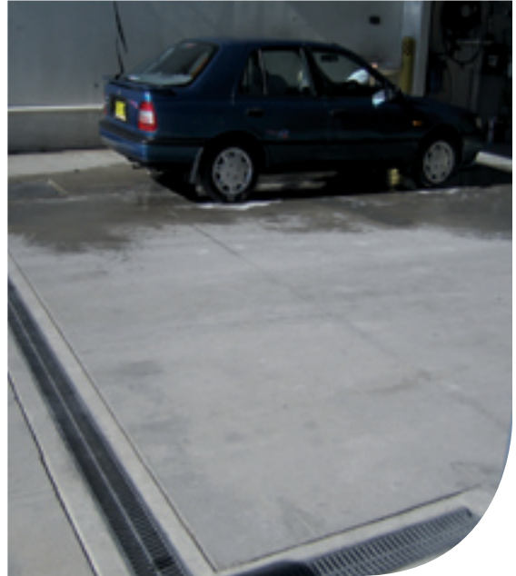
Grated drains ensure that surface runoff and spills are collected in a pit.
